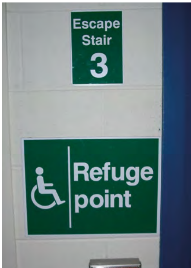
Refuge clearly signed (The Torrent Complex, Donaghmore)
