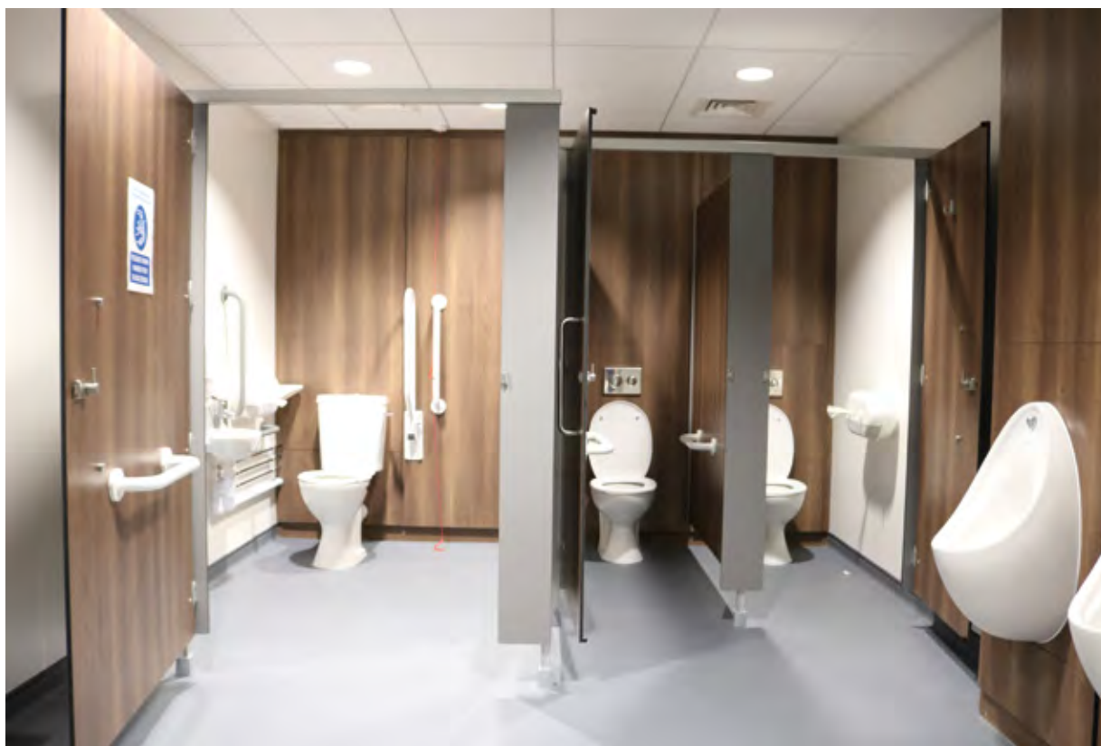
Wheelchair accessible WC cubicle and ambulant accessible WC cubicle incorporated within inclusive toilet block (South Lake Leisure Centre)
