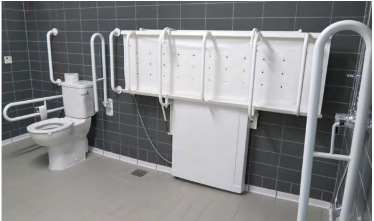
Height adjustable adult-sized wall-mounted changing bench (Newry Leisure Centre)
