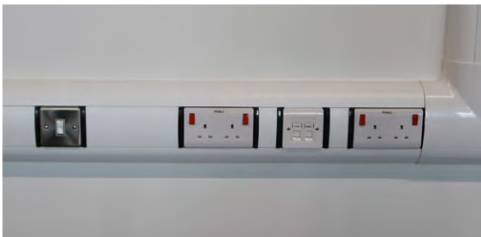
Outlets and switches showing visual contrast (South Lake Leisure Centre)
