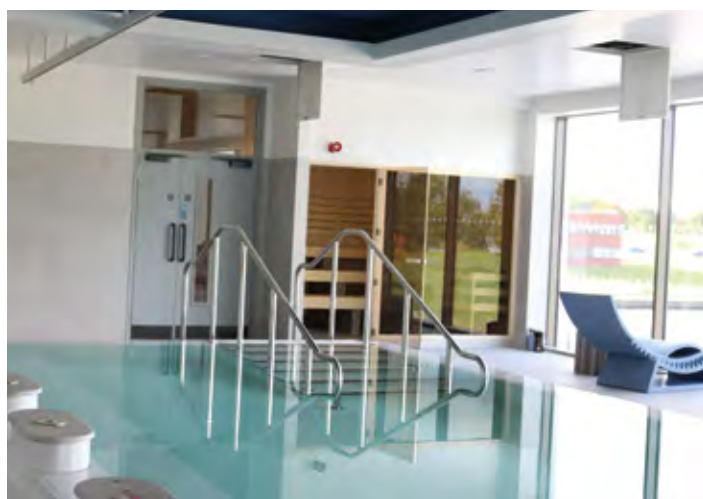
Ceiling tracked hoist provision and steps with handrails and contrasting nosings to vitality pool (South Lake Leisure Centre)
