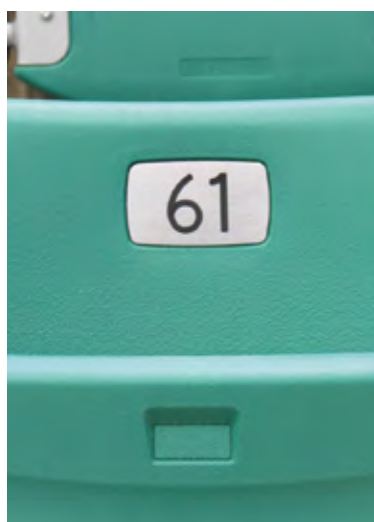
Large contrasting seat numbers (Foyle Arena, Derry~Londonderry)
