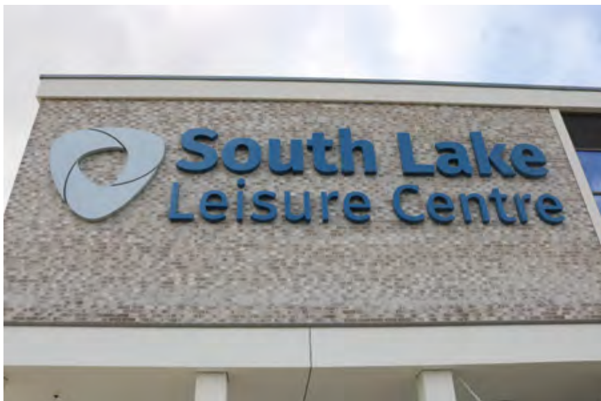
Large facade sign to clearly denote facility name from long distance (South Lake Leisure Centre)
