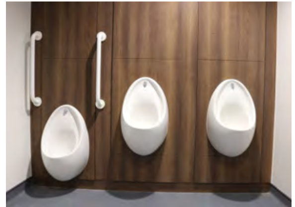
Lowered wash hand basin and urinal provisions, including contrasting grabrails, within inclusive toilet areas (Foyle Arena, Derry~Londonderry and South Lake Leisure Centre)
