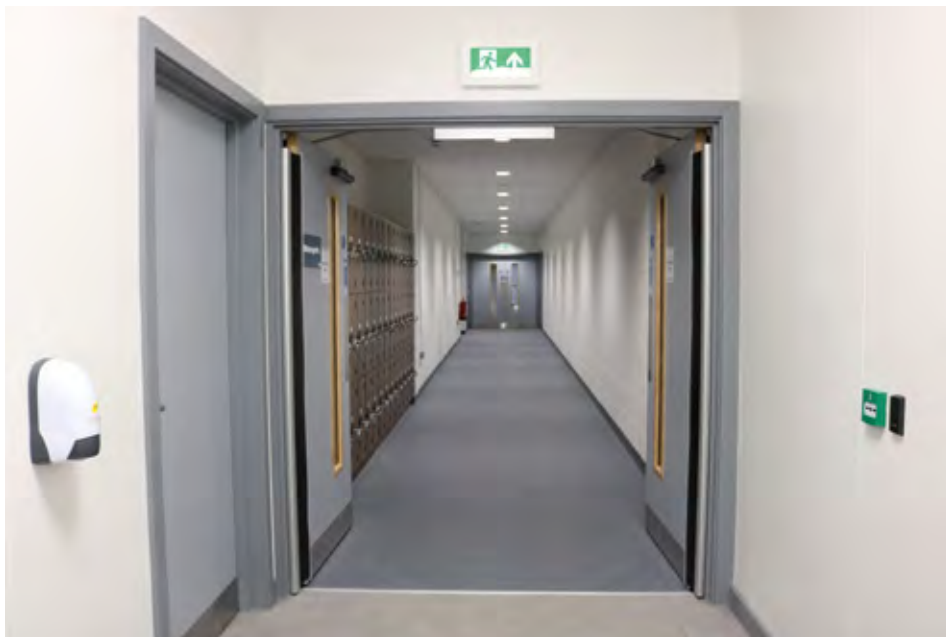
Wide unobstructed corridor circulation and doors fitted with hold-open devices (South Lake Leisure Centre)
