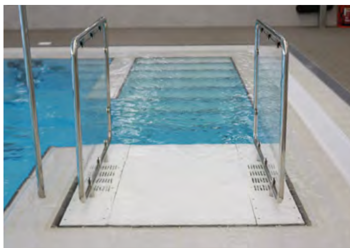
Submersible pool platform and easy steps adjacent (South Lake Leisure Centre)
