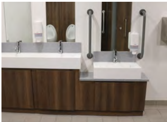
Lowered wash hand basin and urinal provisions, including contrasting grabrails, within inclusive toilet areas (Foyle Arena, Derry~Londonderry and South Lake Leisure Centre)
