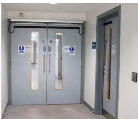
Internal doors showing ironmongery, signs and contrasting trims (South Lake Leisure Centre)
