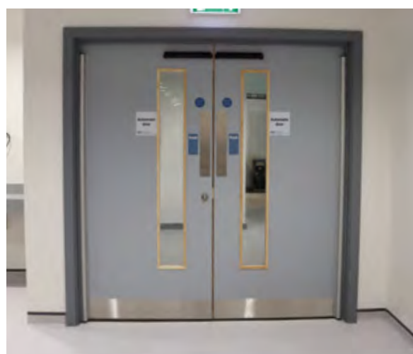
Internal doors showing ironmongery, signs and contrasting trims (South Lake Leisure Centre)
