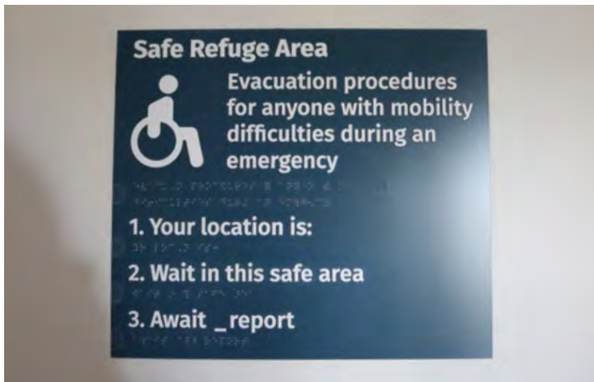
Egress refuge area sign with embossed lettering and Braille (South Lake Leisure Centre)
