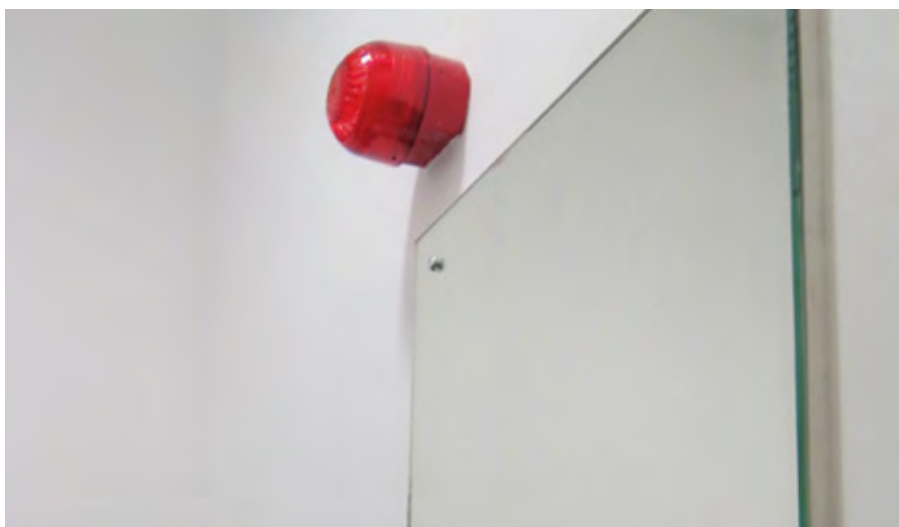
Use of flashing beacon alert within self-contained unisex wheelchair accessible WC unit
