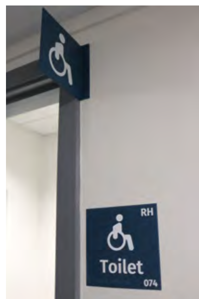
Unisex wheelchair accessible WC signs, including tactile symbols, lettering and Braille (South Lake Leisure Centre)
