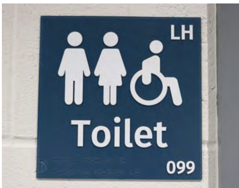
Unisex wheelchair accessible WC signs, including tactile symbols, lettering and Braille (South Lake Leisure Centre)
