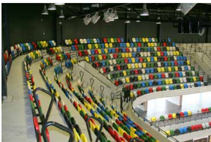
Image 2 - Handholds to Gangways in London 2012 Handball Arena® (image courtesy of Populous)
