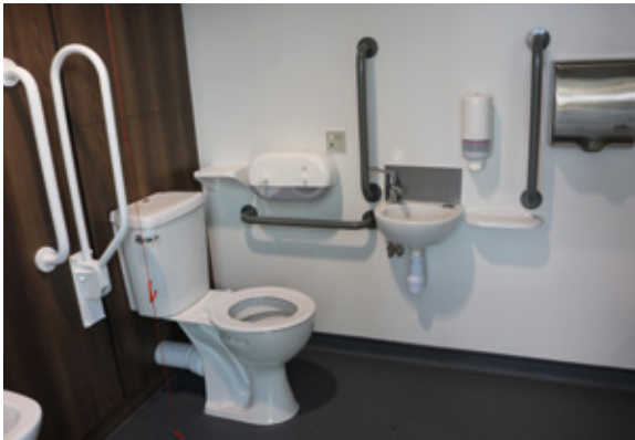
Image 4 - Examples of self-contained unisex wheelchair accessible corner layout WC for independent use
